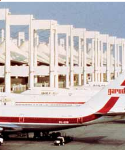
Fig. 1: Walter Bird (with hat) and the architect, John Shaver, inside the Center in 1993 when the structure's 20th birthday was celebrated. Photograph taken by the author. Below: (Fig. 2) The Haj Terminal of 1980 is still the largest fabric structure ever built. Photograph courtesy of Taiyo Birdair Inc.
