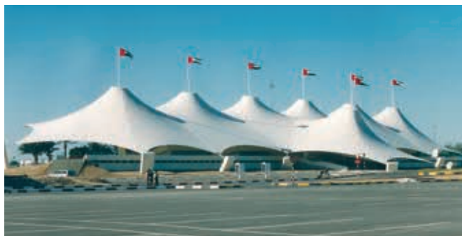
Ladies Pavilion - Abu Dhabi, UAE Précontraint 1202 Fluotop T - Installation: 1996 - Sampling: 2006 Average relative humidity: 65%
