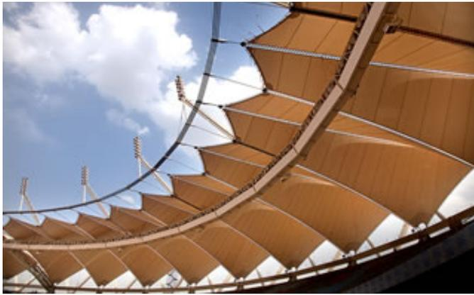
To provide unobstructed views for stadium patrons, a steel compression ring weighing more than 8,500 tonnes and extending 71 meters over the stands supports the tensile roof's [cable net system](#) and PTFE SHEERFILL panels without any perpendicular support from inside the stadium. The cable net system features 443 tonnes of pre-stretched cables with a length of 2,220 km in varying diameters, from 40 mm to 95 mm.
