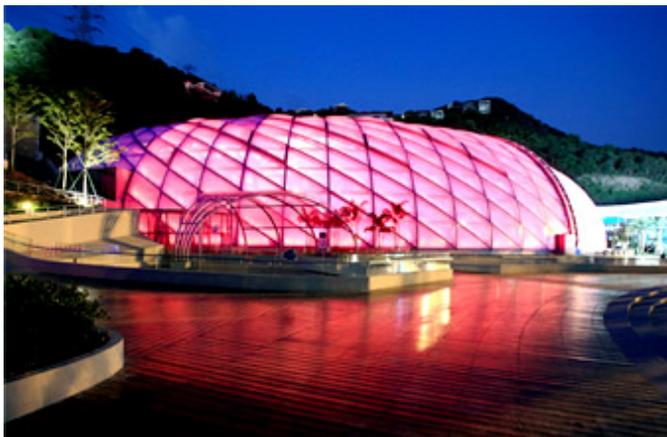
ETFE film can be used in place of traditional glass and plastic for permanent or temporary structures, allowing roof or wall weight to decrease drastically. The material does not shatter upon impact and architects are using ETFE in place of glass in applications where blast mitigation is a concern. When ETFE film is used in a two- or three-
