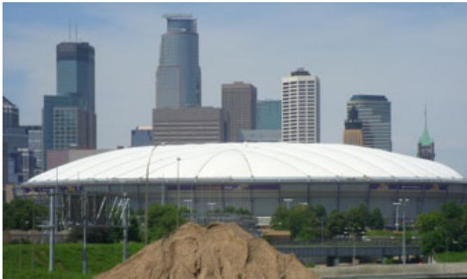
Birdair installed the Metrodome's original roof in 1982 and replaced the structure's 10-acre roof with more than 700,000 square feet of [PTFE-coated fiberglass](#) outer and liner membrane material. The new roof looks similar to the old roof, but features a lower profile.
