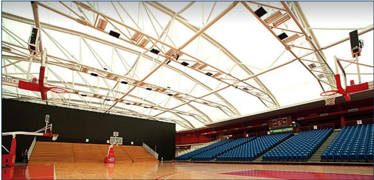
Birdair's first [Tensotherm™ with Nanogel®](#) project provides [thermal efficiency](#) for a roofing retrofit at the Dedmon Athletic Center at Radford University, Radford, Va.
