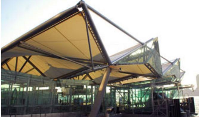
Tensile architecture is a cost-efficient option for projects of any size. Once installed, tensioned membrane structures retain their brilliance over time, with a high level of resistance to staining, soiling and moisture. Fabric membrane roofing systems also offers energy efficiency benefits by delivering high solar reflectance and low thermal emittance values, and by promoting [natural daylighting](#), which reduces reliance on electric lighting.
