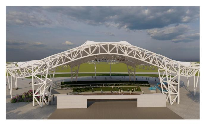
Birdair's scope for the Imagine Clearwater Amphitheater includes design, engineering, fabrication and installation of the main structural steel, fabric roof, cables, catwalks and attachment hardware.
