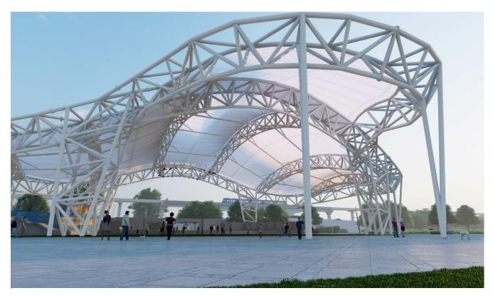
Birdair's tensioned membrane roof at the Imagine Clearwater Amphitheater will feature  $\mathsf{Tensotherm}^\mathsf{TM}$ , a translucent acoustical tensile fabric roofing material.
